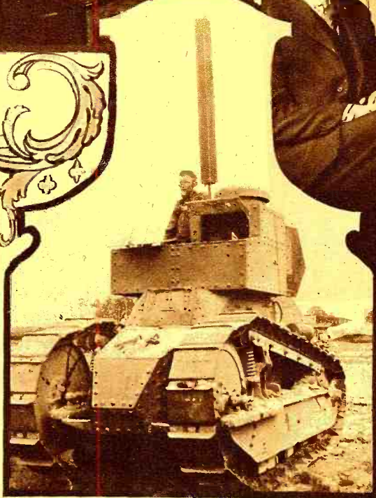
At Left: A "Baby" Tank, Equipped With Radio, is the Newest Instrument of Warfare. The Tanks Are Not Armed, But are Used as a Medium of Communication Between the Front Line and Headquarters. The Special Aerial is Placed on Top of the Tank, Which is Manned by a Driver, and a Radio Operator.
