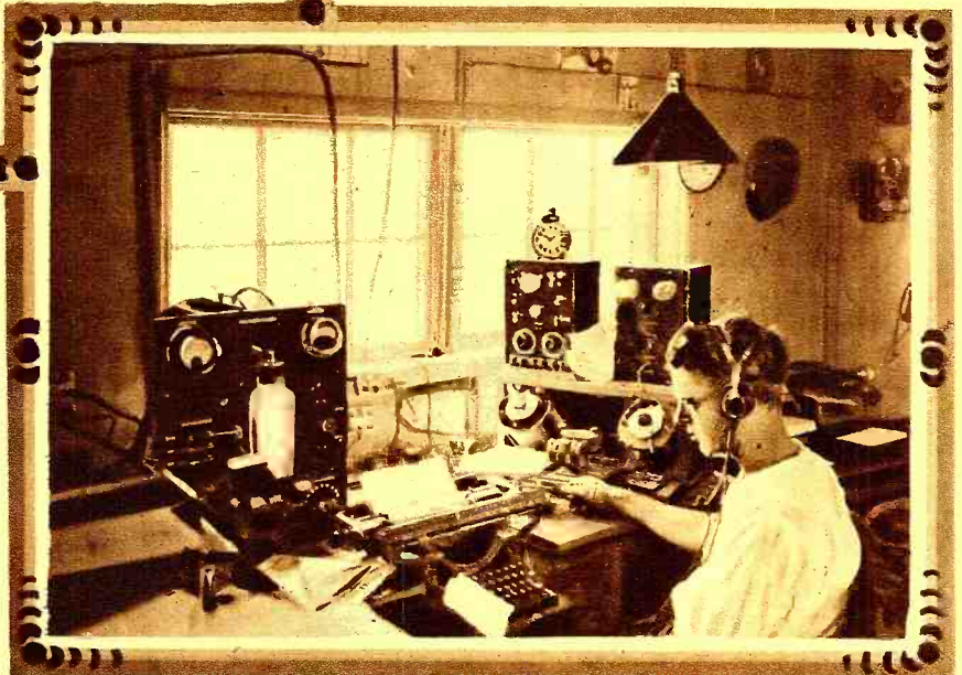
The Radiophone Station Installed by the Southern California Edison Co. to Keep in Touch With the 500 Men Working on a Tunnel in the Mountains.
